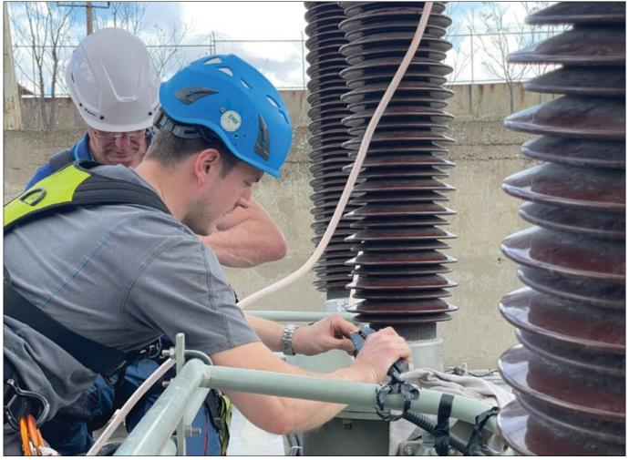
Figure 8. Installation of bushing sensors for the HYDROCAL BPD
